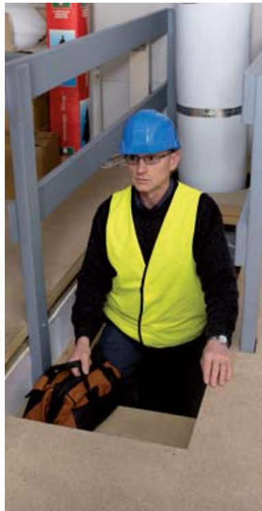
Flooring platform between the roof and ceiling for extra storage.
